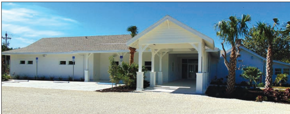
The Community House's new eastern entrance contains a covered drop-off area photos by Jeff Lysiak
